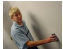
Corey Rittenhouse sands drywall at FCCI.
